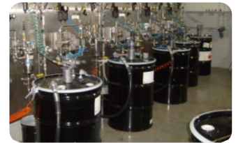
PAINT CIRCULATING SYSTEMS
